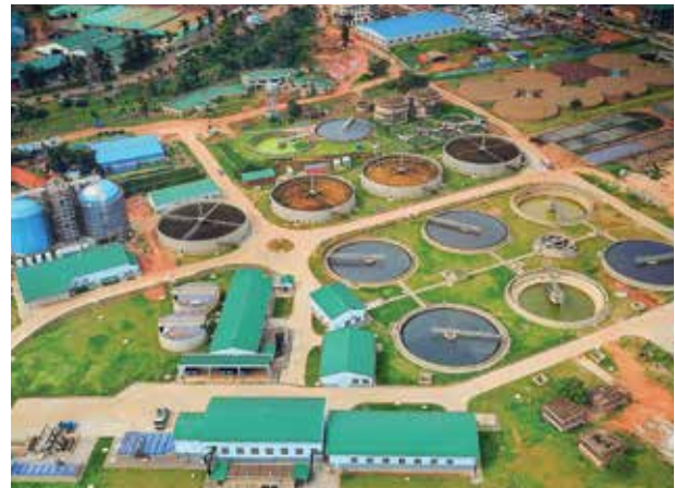
Nakivubo Wastewater Treatment Plant - Bugolobi
