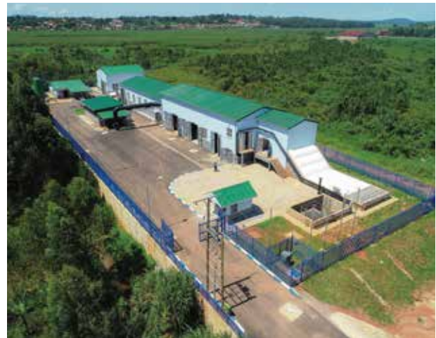
Kinawataka Wastewater Pre-Treatment Plant
